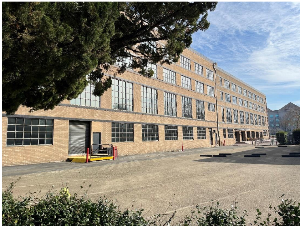
Photo 4. South elevation, view northeast from RS Alley.
