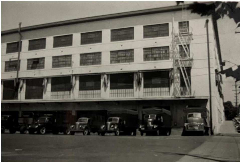
Figure 4. Recessed truck loading bays at the south elevation, ca. 1946. Source: Center for Sacramento History.
