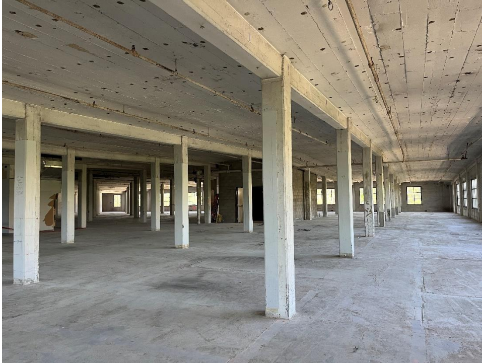
Photo 21. Fourth floor, original 1911 building, view north, typical.
