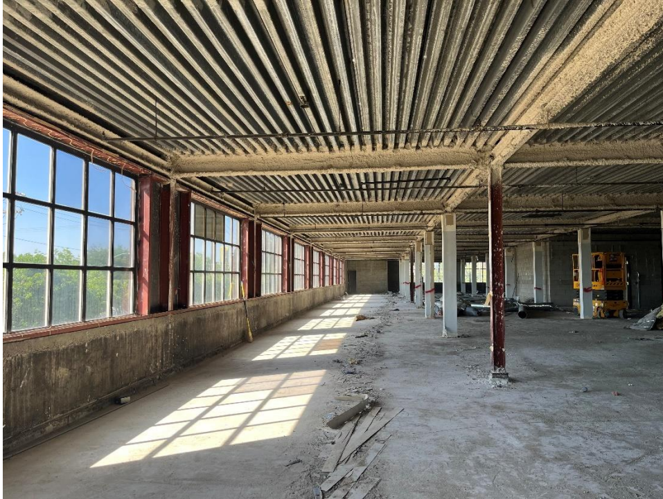
Photo 19. Third floor, 1947 addition, view north, typical.
