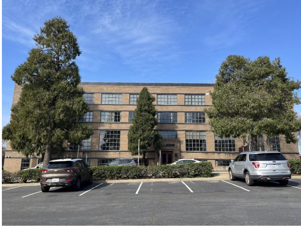
Photo 1. East facade, view west from surface lot on opposite side of 3rd Street.
