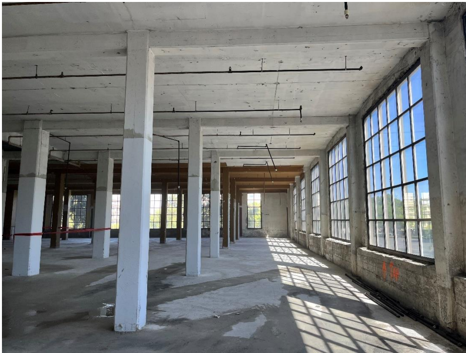
Photo 14. Second floor, original 1911 building, view east, typical.
