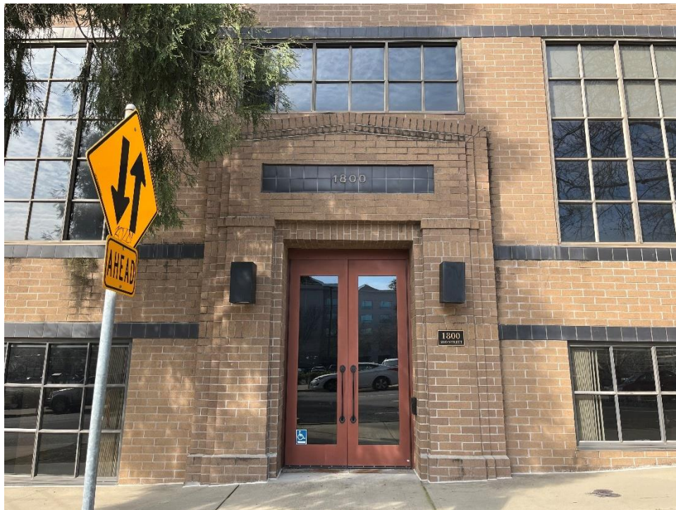
Photo 2. East facade, historic main entrance at center of facade; view west.
