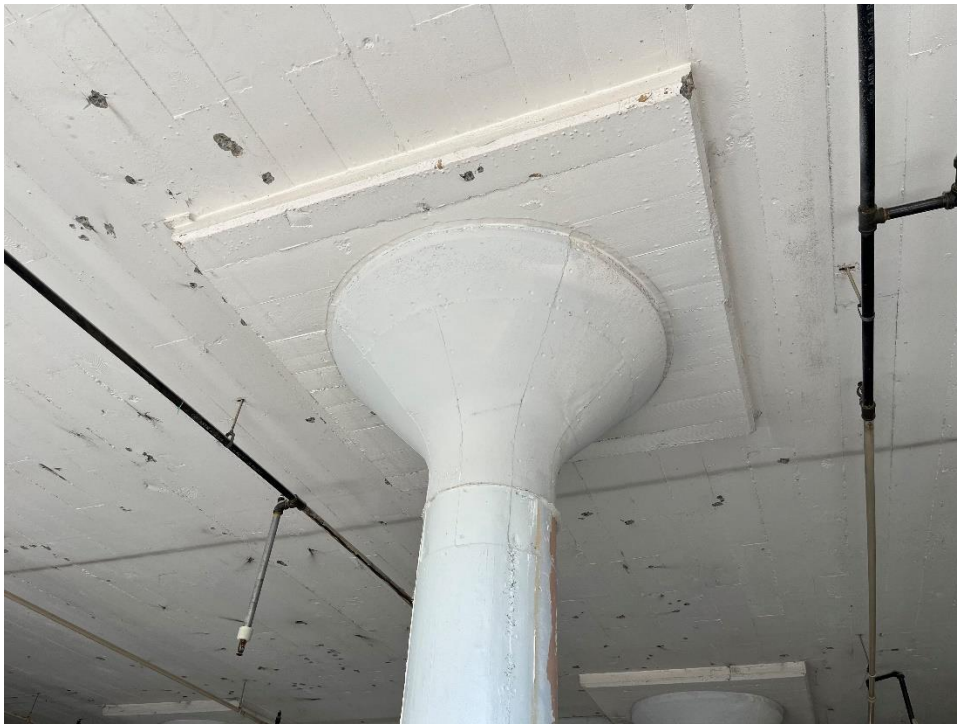
Photo 12. First floor, 1936 west addition, detail of mushroom column capital, typical.
