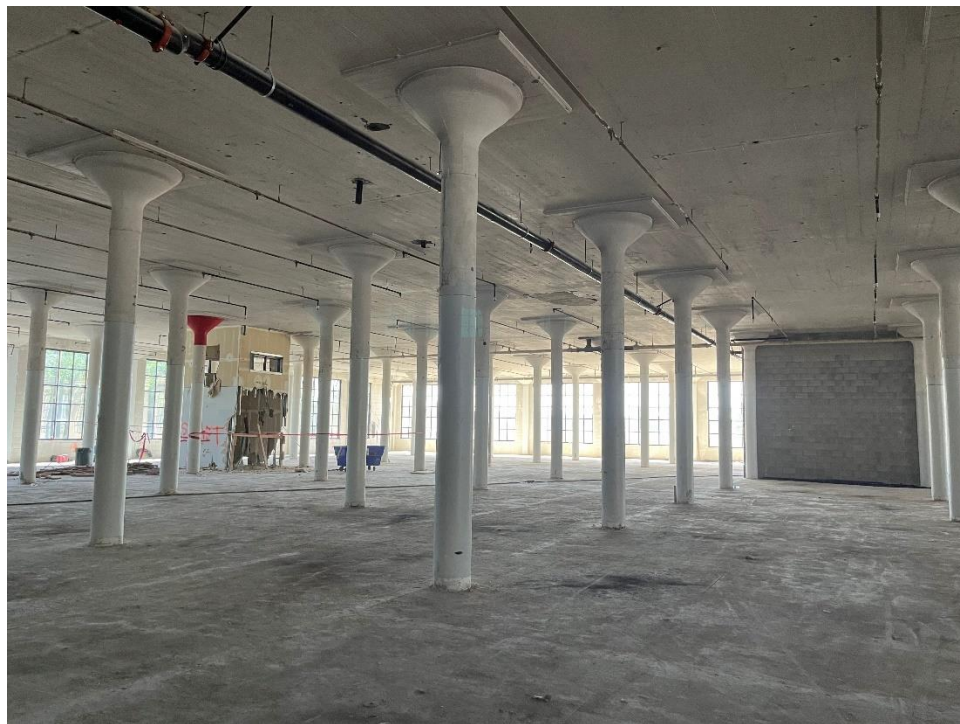
Photo 16. Second floor, 1936 west addition, view southwest, typical.
