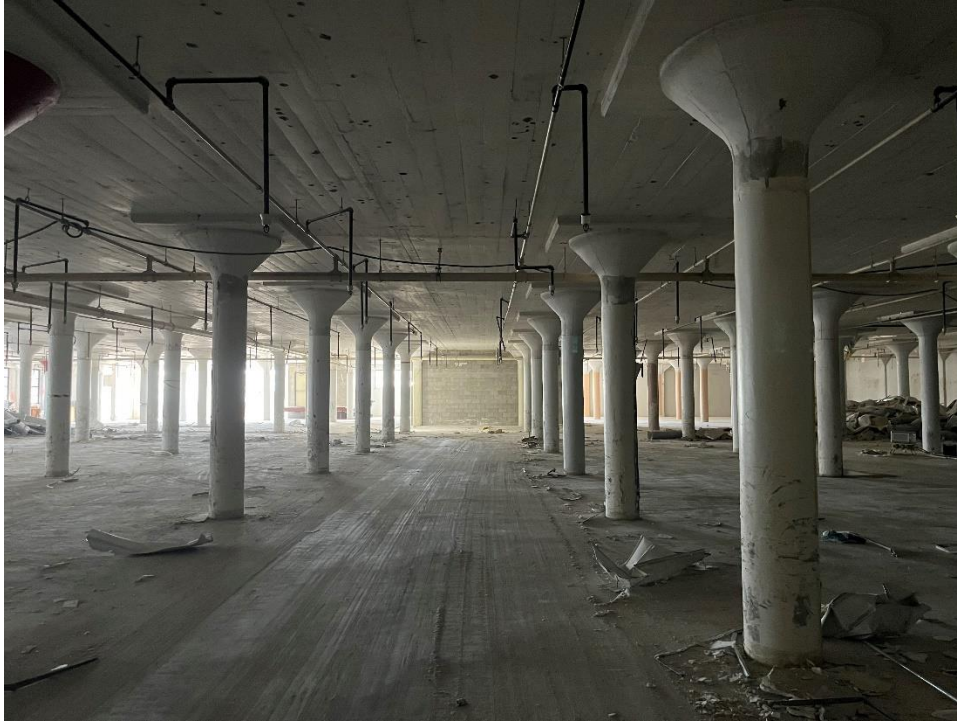
Photo 11. First floor, 1936 addition, view west, typical.
