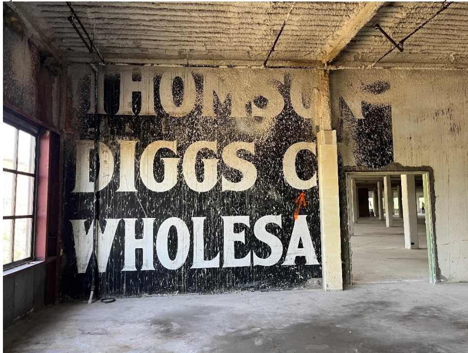
Photo 23. Fourth floor, 1947 addition, top of "Thomson Diggs Co. Wholesale Hardware" ghost sign on demising wall between the 1911 and 1947 portions of the building, view east.
