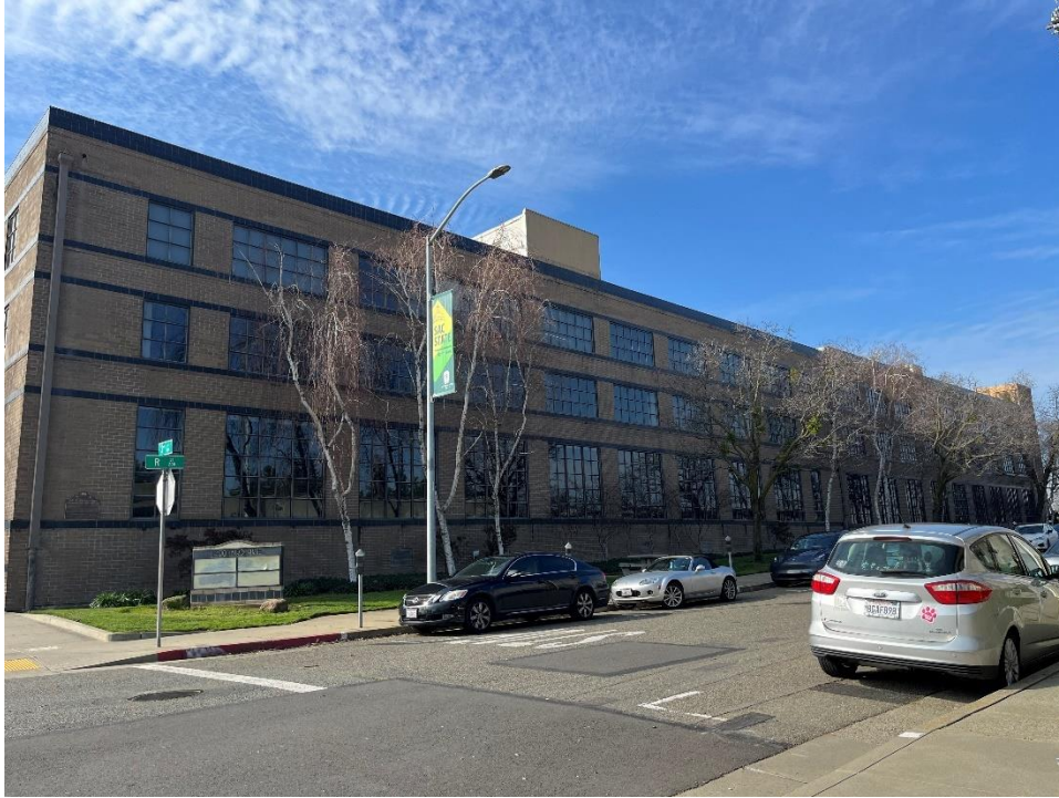
Photo 7. North elevation, view southwest towards monument signage.
