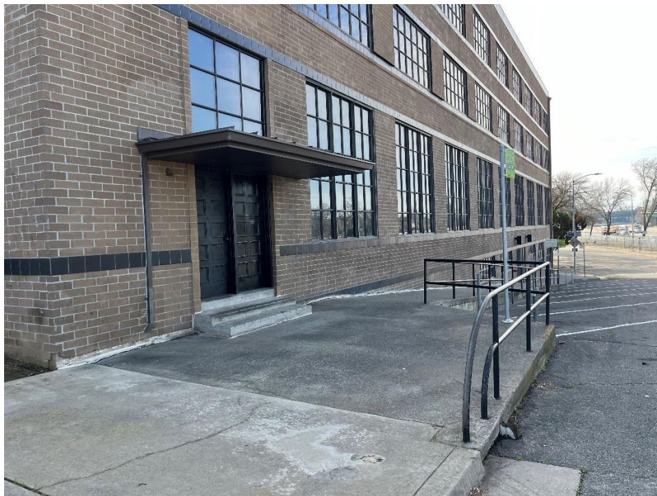
Photo 6. West elevation, historic entrance into West Addition with paneled metal doors and curved metal pipe railings, view south.
