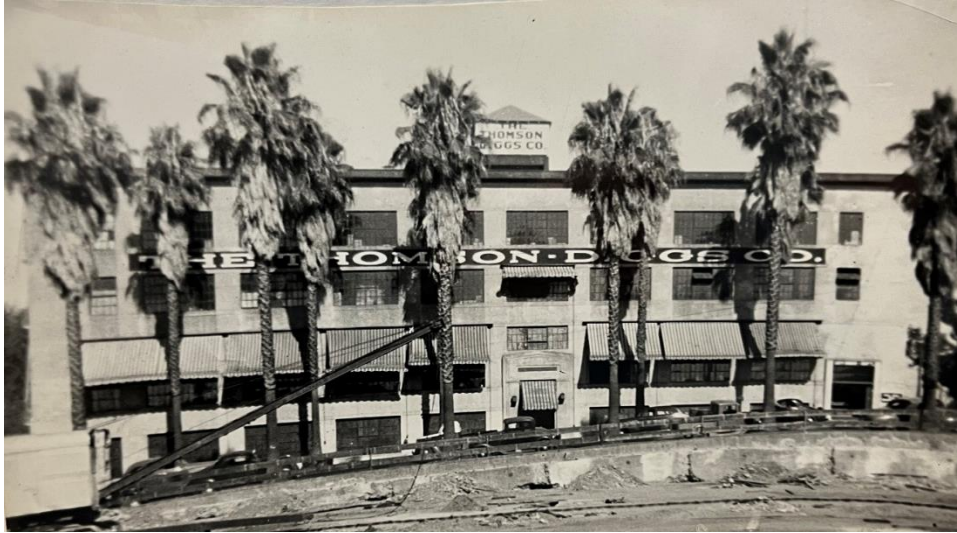
Figure 3. The east facade, view west, undated. Source: Center for Sacramento History.
