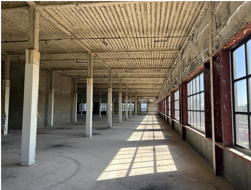
Photo 22. Fourth floor, 1947 addition, view south, typical.
