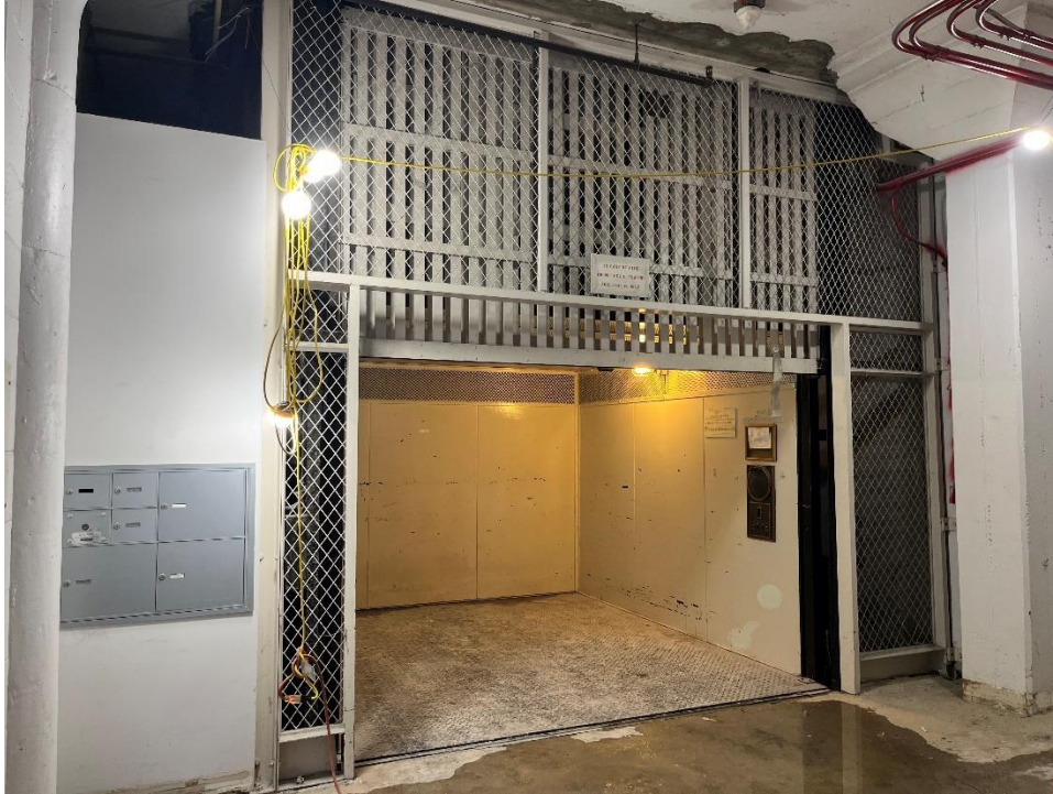
Photo 13. First floor, 1936 west addition, historic freight elevator at southeast corner.
